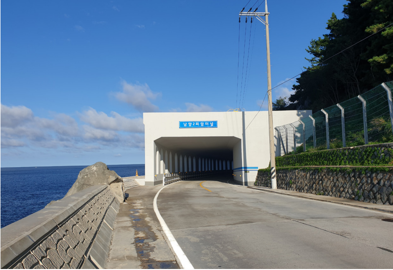
Namyang No. 2 Rockfall Protection Tunnel photographed on October 1, 2023
