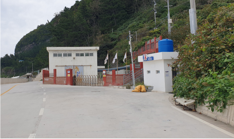
Hydroelectric Power Plant photographed on October 2, 2023
