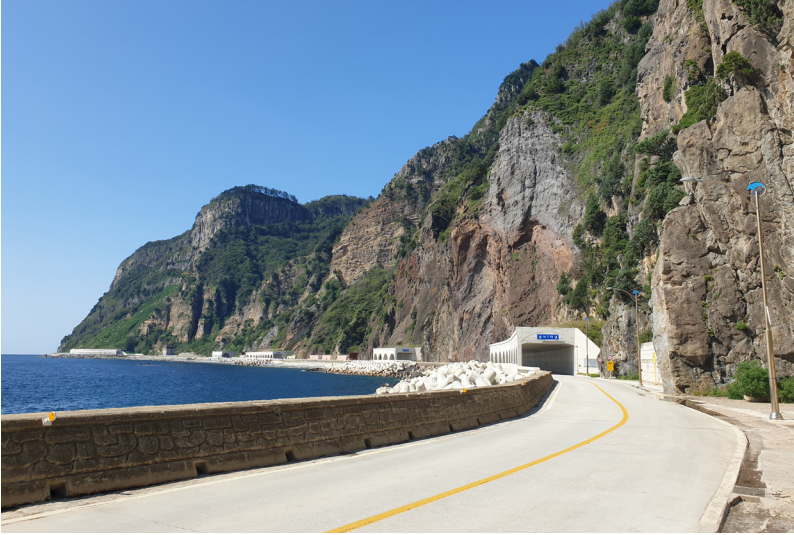
Namseo Tunnels 2, 3, 4, and 5 photographed on October 2, 2023
