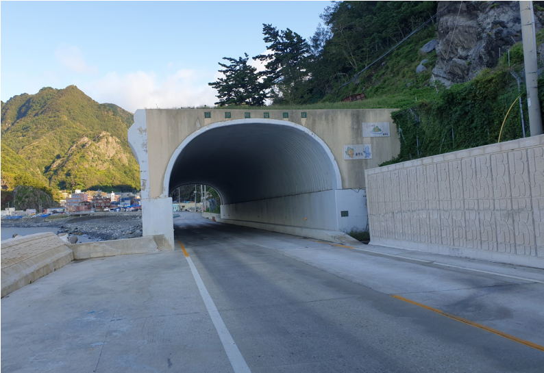
Namyang Rockfall Protection Tunnel photographed on October 1, 2023
