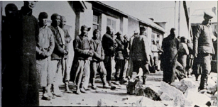
威海卫华工营内等候体检的华工 (摄于1917年) Chinese laborers waiting for physical examination in Weihai Port Chinese Laborers Camp (photo taken in 1917)
