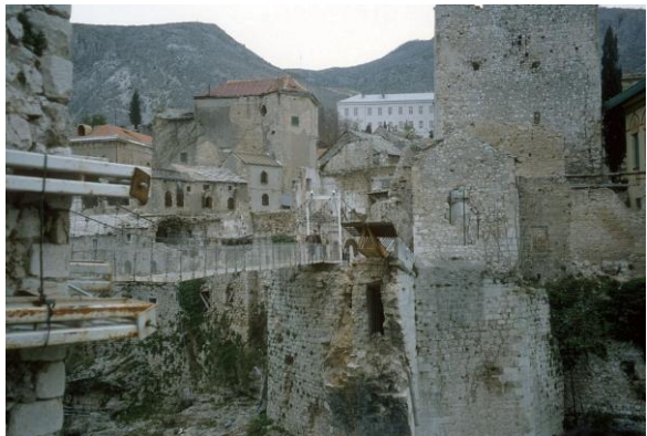
Temporary bridge installed in 1993 after destruction (Source: https://commons.wikimedia.org/wiki/File:Stari_Most_temporary_cable_bridge_1997.jpg )
