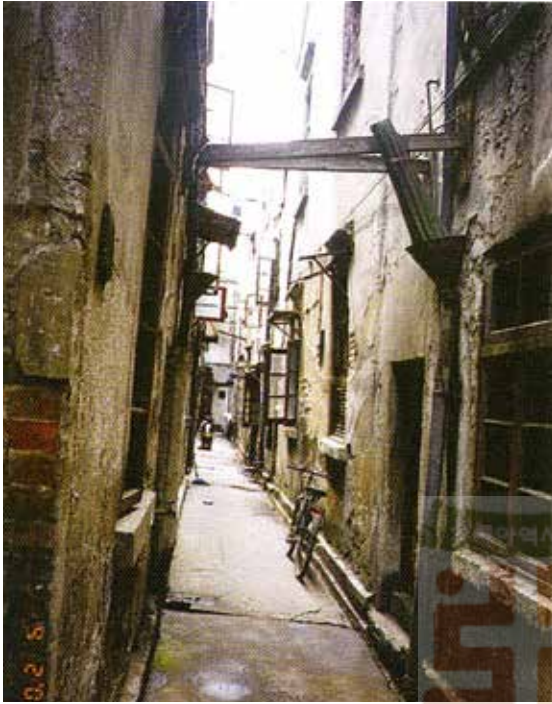
The old site of a comfort station in Jiqingli, Hankou, China
