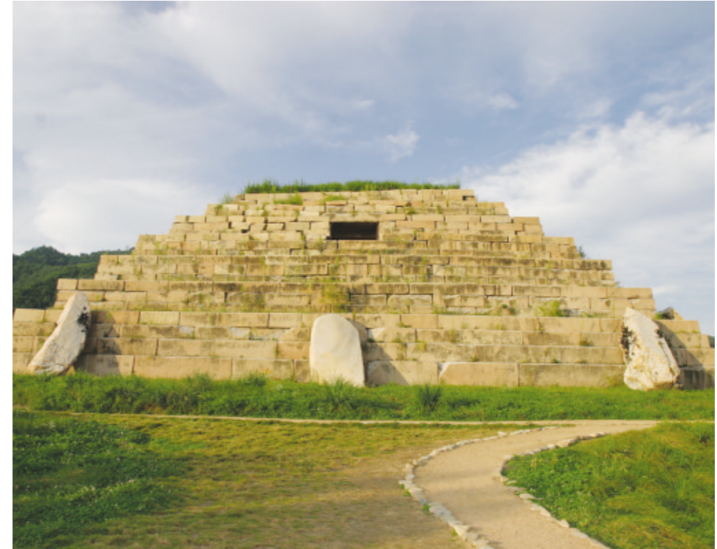
General's Tomb, 5th century (At Ji'an City, Jilin Province, China) Here is a classic example of the stair-shaped stone mound tomb from Koguryo. The structure is almost completely intact after more than 1,600 years, testimony of the construction skills of the Koguryo people.
