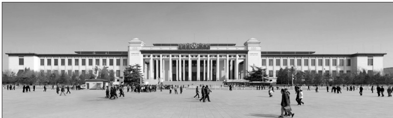
Figure 5. The restored west façade with the staggered roof of the new building, courtesy of Christian Gahl 2011
