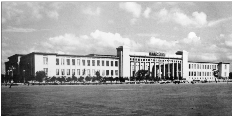
Figure 2. The original West Façade (1959), from Beijing shida jianzhu sheji , 2002, 166
